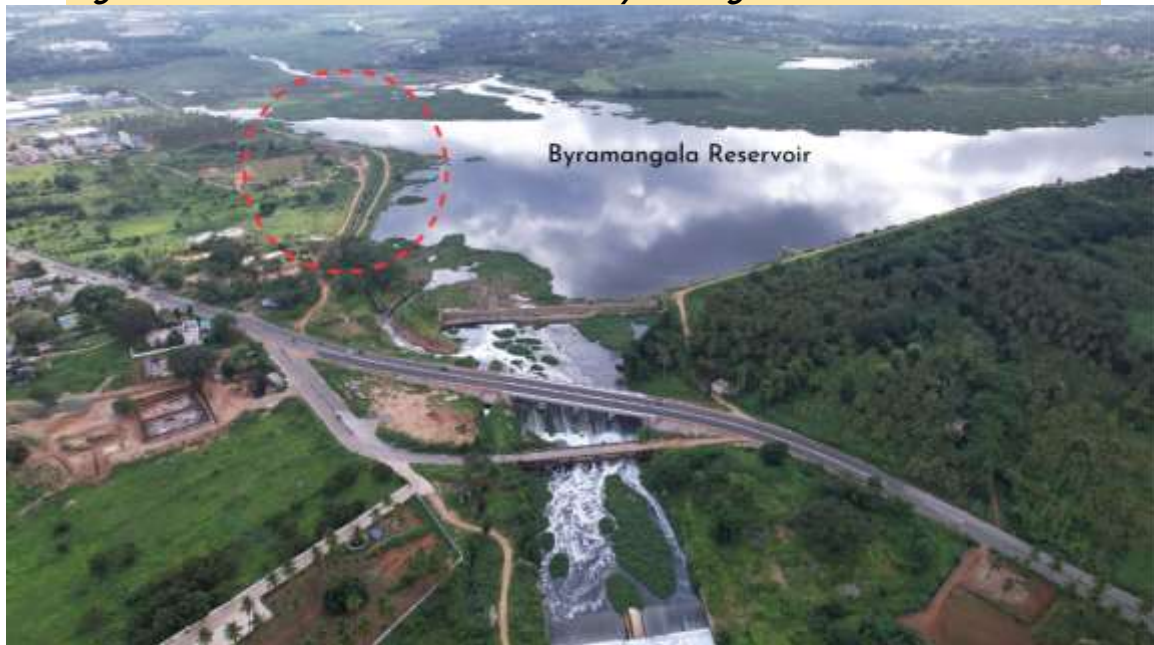
Figure 20: Concrete Channel Built for Byramangala Reservoir Restoration
