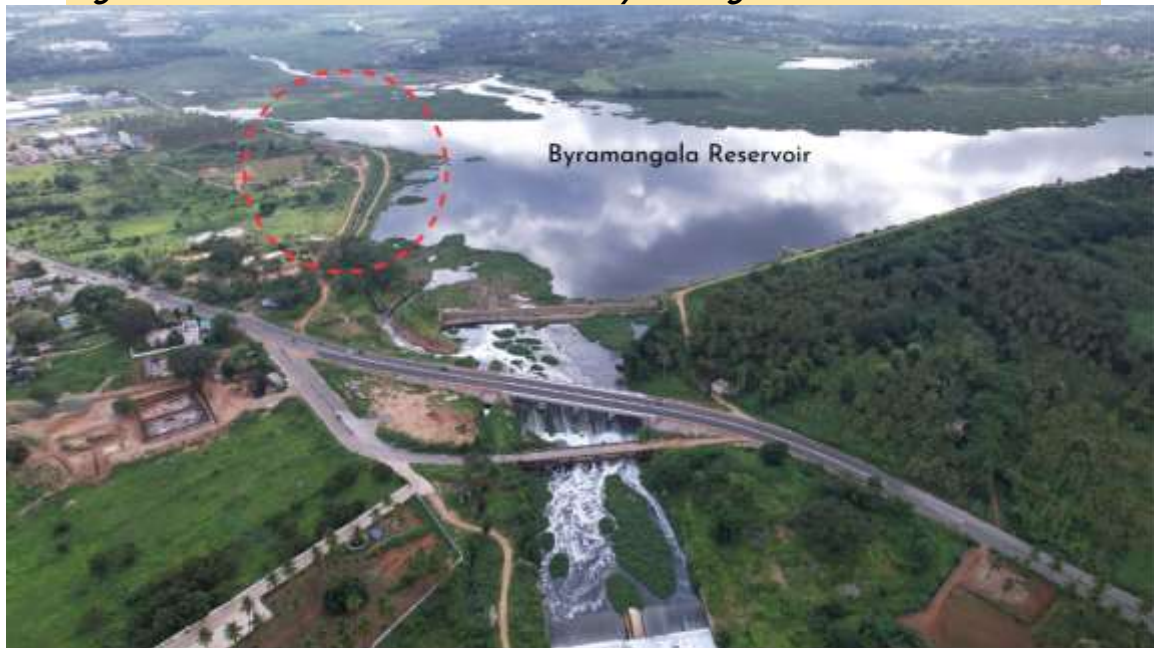
Figure 20: Concrete Channel Built for Byramangala Reservoir Restoration
