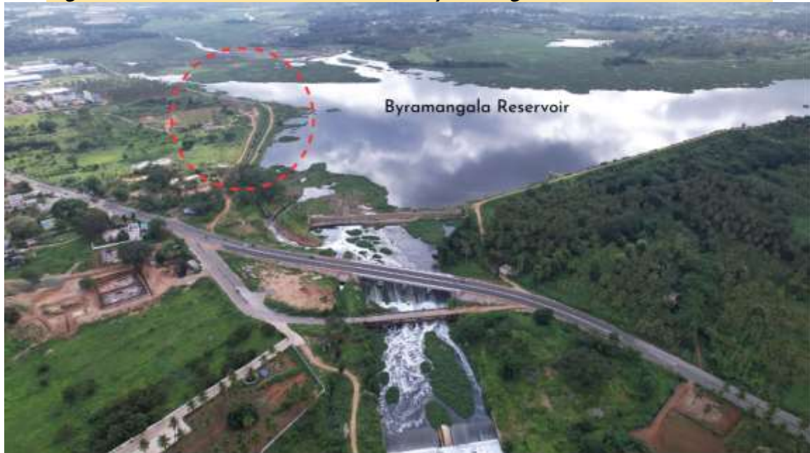
Figure 20: Concrete Channel Built for Byramangala Reservoir Restoration
